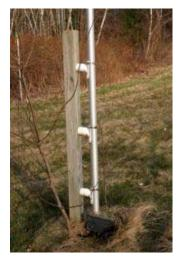
Chet Slabinski, N8RA, recently ran the 7/8 hardline he got from me out to a junction box at one of his towers. To seal the entrance into the box, Chet found that plumber's putty was easy to use and made a good watertight seal.
